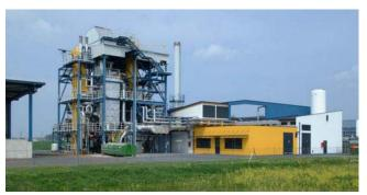
biomass, through a biomass gasifier coupled with an Internal Combustion (IC) gas engine with an electrical efficiency of 25% and a heat efficiency of almost 50%. The gasification plant produces 4.5 MW of heat for the local district heating network.<sup>6</sup>
